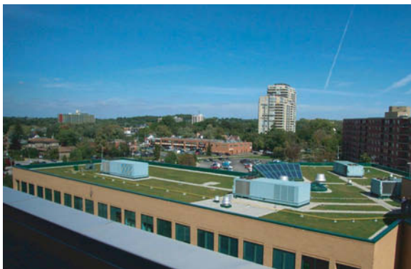
FIGURE 6-3 GREEN ROOF ON CITY OF WATERLOO MUNICIPAL BUILDING, WATERLOO, ONTARIO
