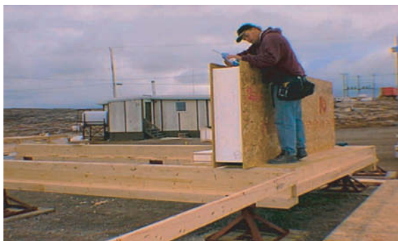
FIGURE 7-18 BUILDING WITH STRUCTURAL INSULATED PANELS (SIPS)
