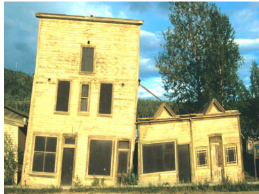
FIGURE 7-17 EFFECTS OF MELTING PERMAFROST ON BUILDINGS IN DAWSON CITY, YUKON
