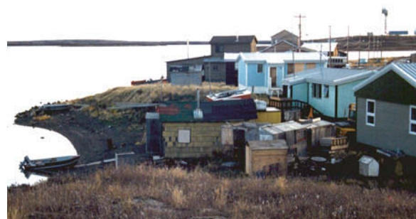
FIGURE 7-4 OLDER HOUSING IN TUKTOYAKTUK, NORTHWEST TERRITORIES
