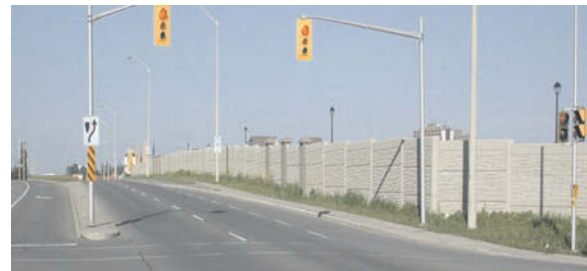
FIGURE 6-11 EXAMPLE OF A NOISE BARRIER
